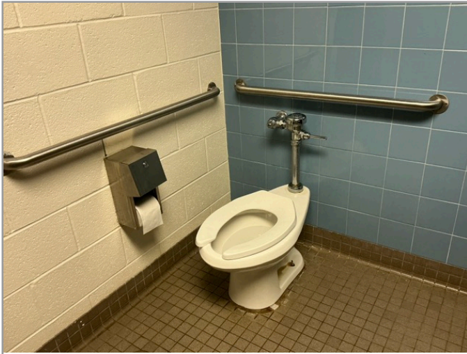
TOILET STALL OVERVIEW
