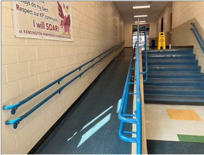
ACCESSIBLE INTERIOR RAMP
