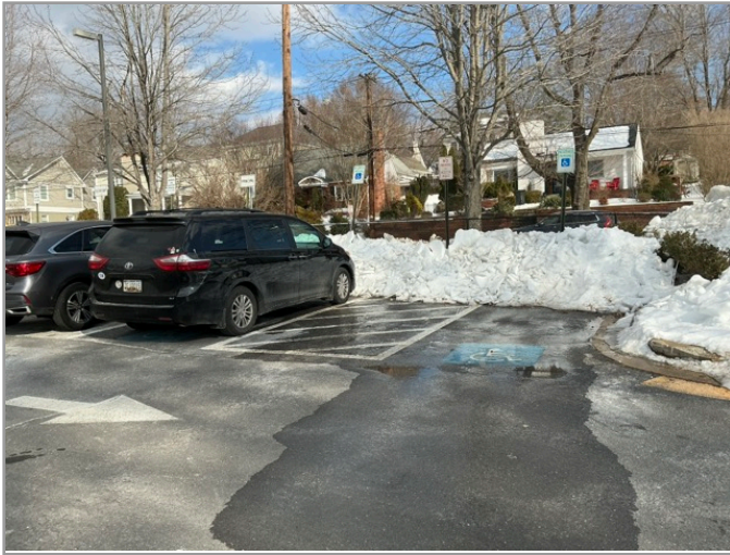
OVERVIEW OF ACCESSIBLE PARKING AREA
